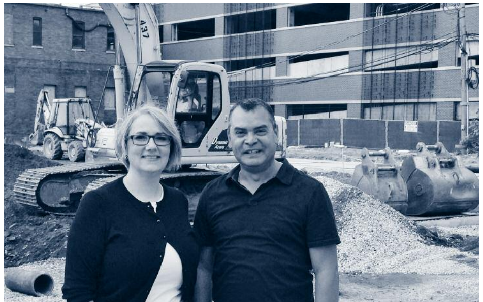
Serena Worthington and Center on Halsted Executive Director Modesto Tico Valle touring the construction site.
